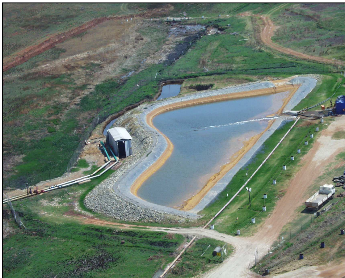
Photo 2 – The dam constructed to intercept water decanting from the Black Reef incline shaft in the Tweelopiespruit. (Photo taken by G. Krige on 05/10/2004)
