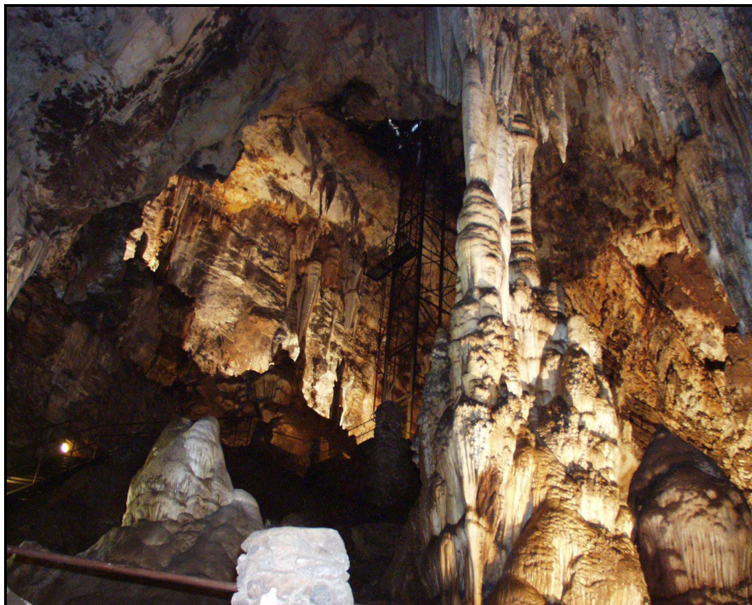
Photo 6 – A section of the Wondercave. Probably only 30% of the void is visible in this photo. The 36-meter lift shaft structure is visible in the centre of the picture. The approximate total void volume of the Wondercave is 240 000 m 3 .
